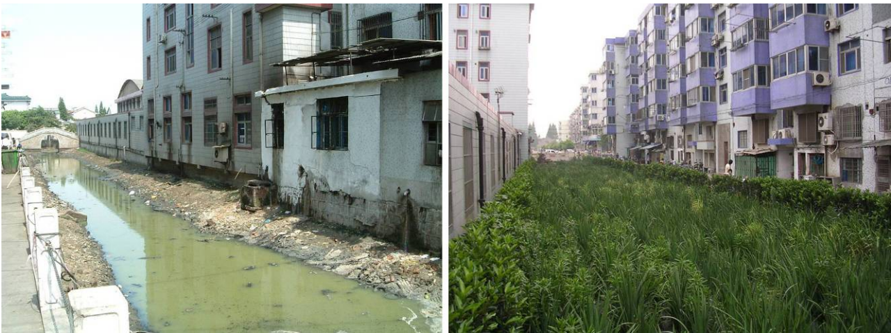
Figure 9: Constructed wetlands to create green and meaningful residential open space in HuaXin, Shanghai (Ingenieurgesellschaft Janisch & Schulz mbH)
